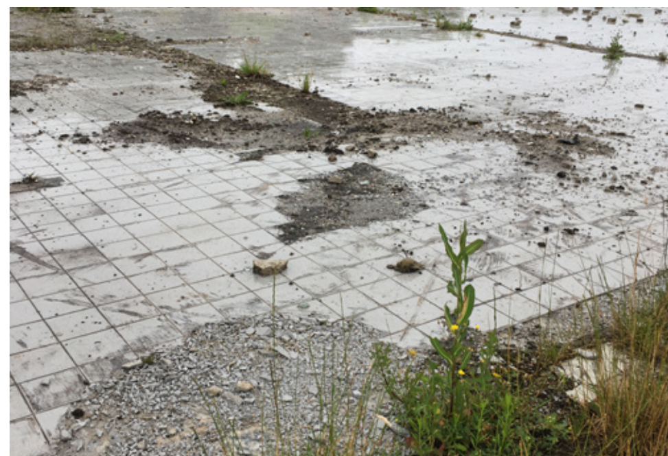
Gaten in de verharding
